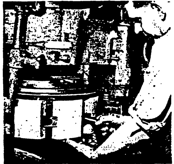
ILLUSTRATION No. 79 A segmental wheel assembly.
