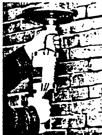
ILLUSTRATION No. 14 Tuck pointing using a reinforced organic bonded grinding wheel.
